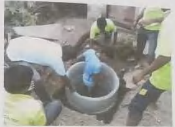
Construction of Toilets
