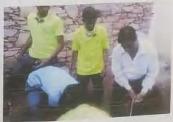
Volunteers Working to Construct Toilets
