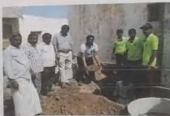
Toilet Construction – Dig the pits . Dr Sangalad & Volunteers
